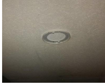
Removed Smoke Alarm
