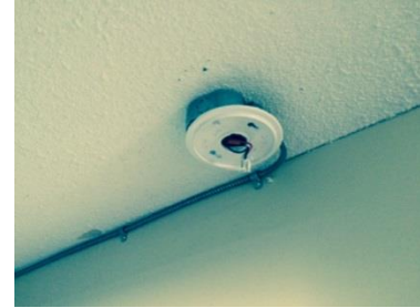
Disabled Hard Wired Smoke Alarm
